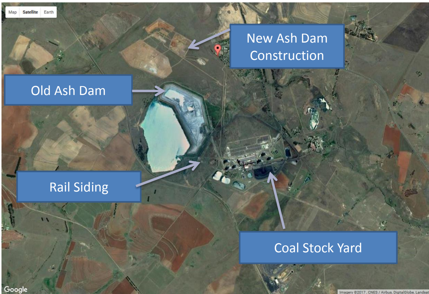
Figure 1: Plants or areas within the facility generating fugitive emissions
